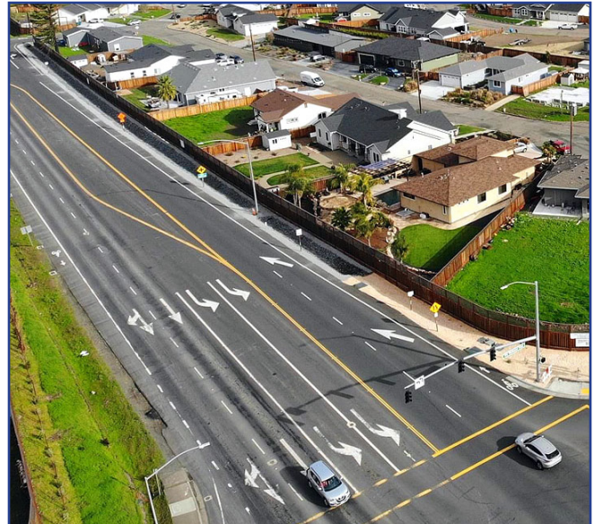
The new sidewalks will improve safety and access for kids and others who walk or navigate wheelchairs along either side of Mark West Springs Road.
