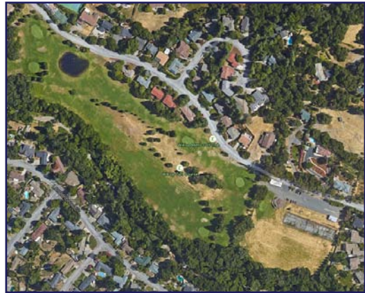
An aerial view of part of the future Wikiup Commons, formerly the Wikiup Golf Course.
